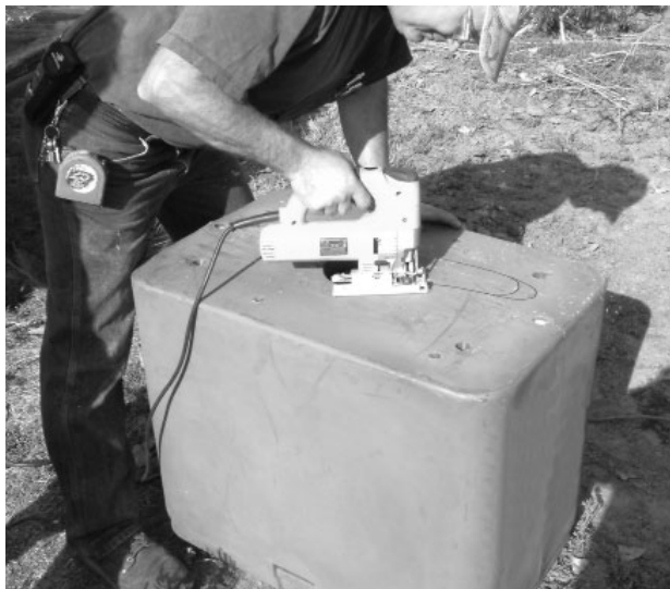
Illustration #2 - Enlarge Hole As Needed
